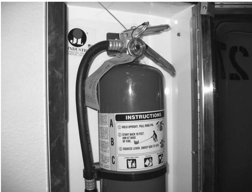
**Figure 4.37** Type A-B-C fire extinguisher
