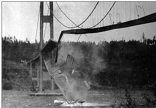
Figure 1 A 600-foot section of the Tacoma Narrows bridge crashes into Puget Sound as the bridge twists and torques itself to death. Mechanical engineers are warned early on that this can happen if they don’t practice good engineering.
