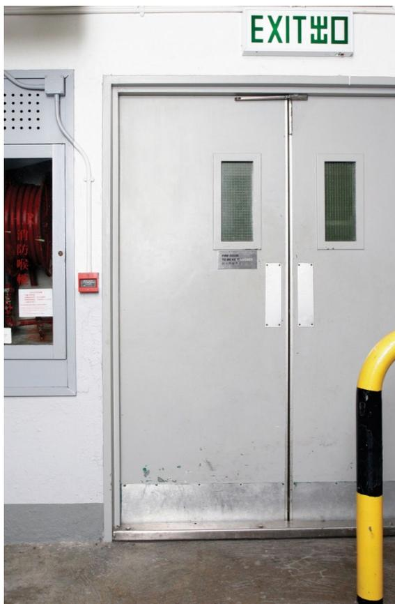
Figure 7-5 A heavy door that can cause a lot of signal attenuation and typically breaks roaming
