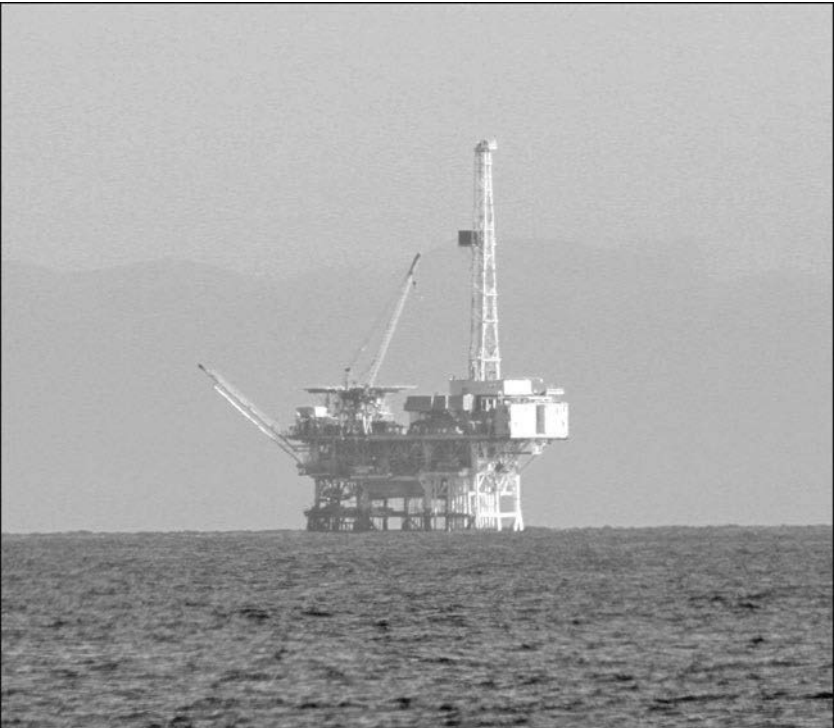
FIGURE 1.1 A modern oil-drilling ocean platform. Platform Holly, a few miles off the coast from Santa Barbara California, was installed in 1966 and has produced oil since. (Source: Linda Krop, Environmental Defense Center, Santa Barbara, CA)
