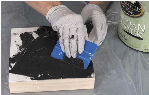
**FIGURE B.7** The black plaster layer doesn't need to be perfectly smooth.
