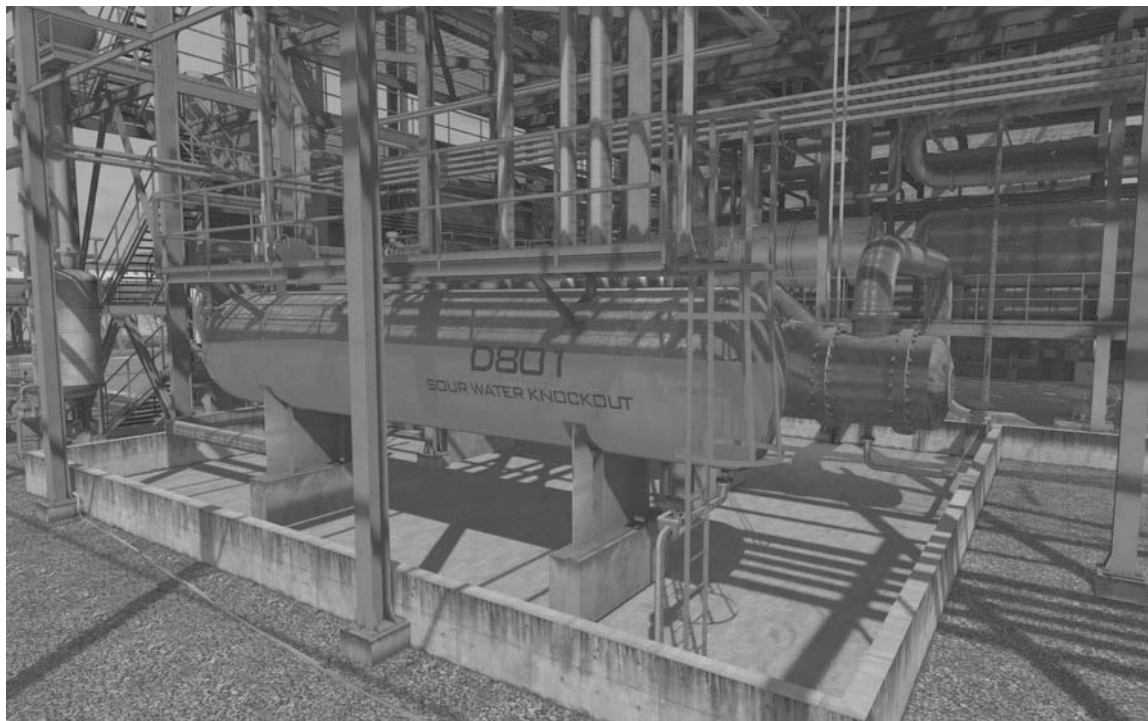
Figure 1.17 An Example of a Computer-Generated Image of a Horizontal Drum (Reproduced by Permission of the DOE's National Energy Technical Laboratory and Invensys Systems Inc., Property and Copyright of Invensys plc, UK)
