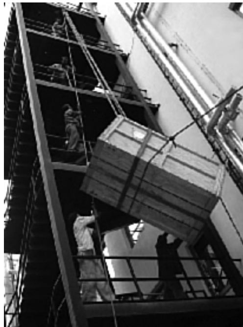
Figure 2-2 Moving Equipment Without a Freight Elevator
