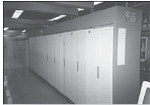
Large Telephone Switches
