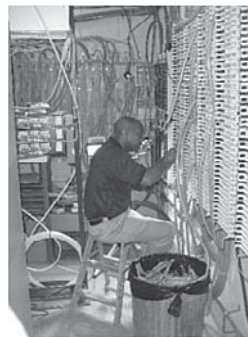
Wiring Closet Infrastructure
