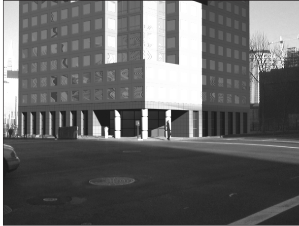
Figure 10.14 Camera Matching 3D buildings against an image of a site. Using points measured from the actual site in the photograph, Camera Matching can compute the original camera's perspective and apply those settings to the camera in your scene for accurate compositing.
